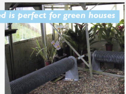
Secondary heating to alleviate down draughts and condensation
